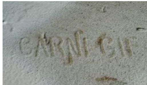
Steel Girder Detail at Nanue Bridge
